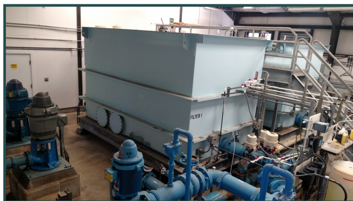
Water District 19 Water Treatment Plant
